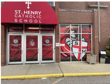
Main entrance to school
